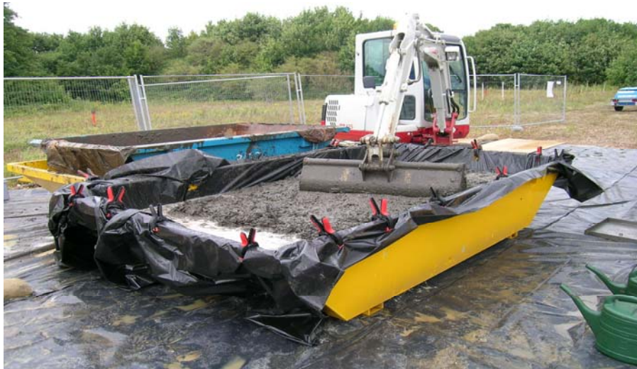
Figure 8. Soil Transfer in Progress
