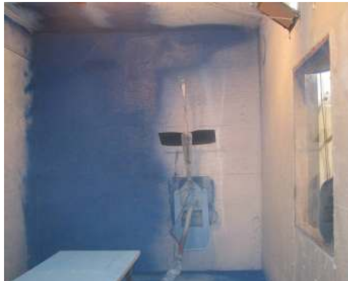
Figure 5. PBS fixative being sprayed on hot cell mockup wall
