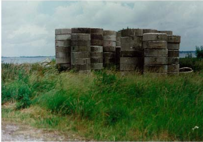
Fig. 1 Storages consisting of stacked concrete rings. The storages contained concrete-lined steel drums filled with a mixture of concentrate from the distillation facility and bitumen.
