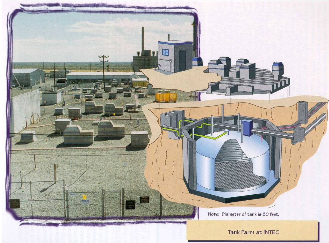
Figure 2. Tank farm to process Spent Nuclear Waste at INL.
