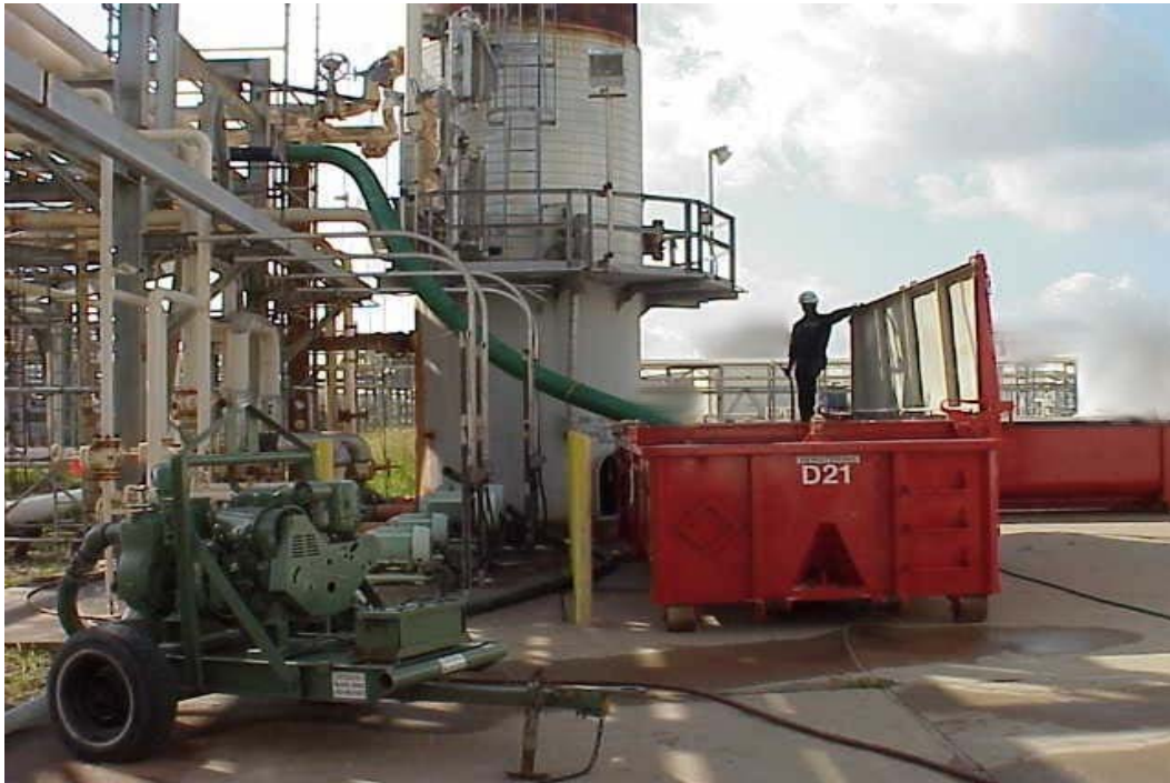
Figure 3. Typical installation of Hydrokinetic™ System.
