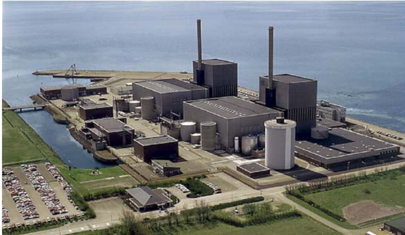
Picture 1 Barsebäck NPP in Sweden
