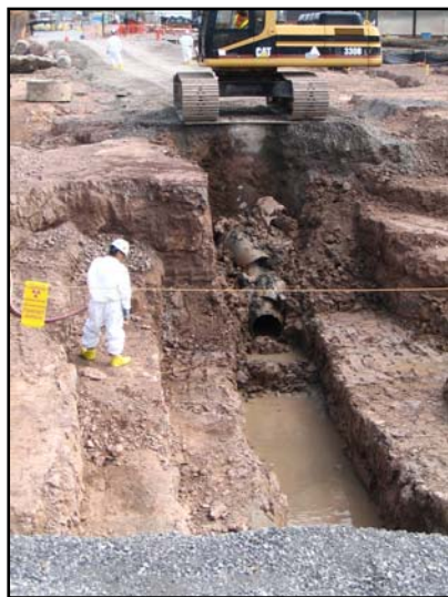
Sewer Line Remediation
