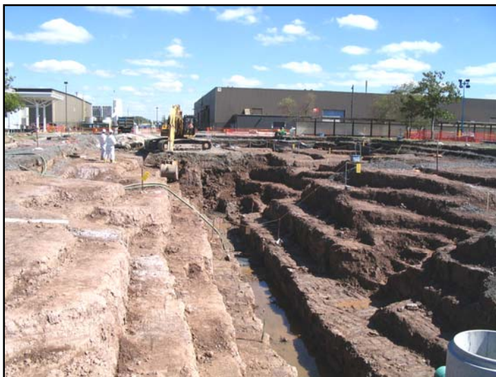
Benching of Excavation Sidewalls
