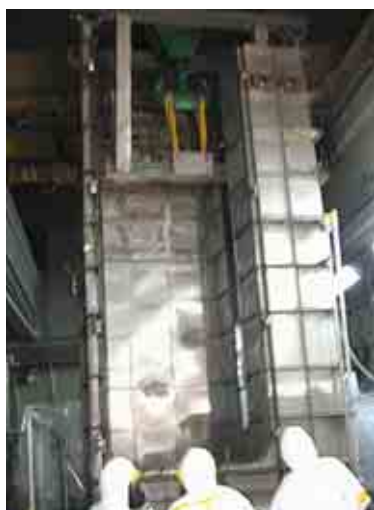
Figure 3. Metal basin 5 m long during extraction from EUREX SFP.
