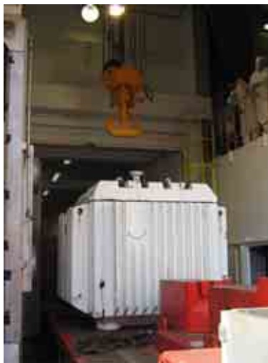
Figure 2. Load test after crane revamping.
