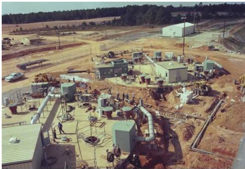
Fig. 1. SRS Tank Transfer Piping Construction
