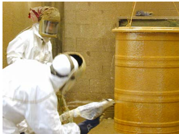
Fig. 2: Finishing of work
