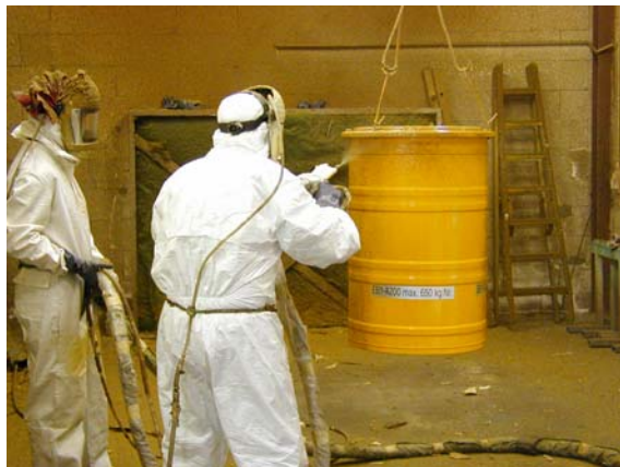
Fig. 1: Coating with Polyurethane
