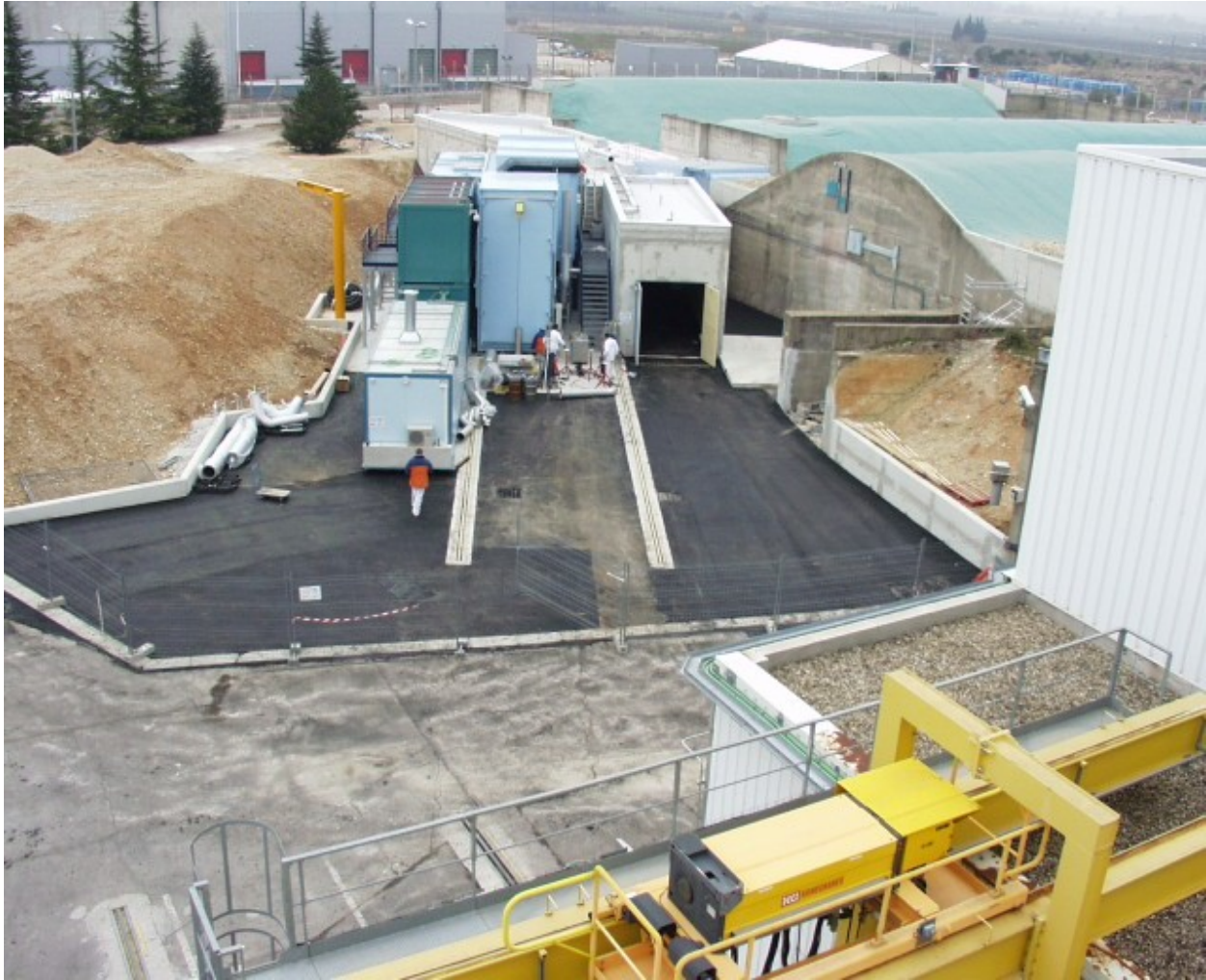
Fig. 2. Photograph of AREVA's second-generation mobile hot cell (ERCF) deployed at the Marcoule Site, France.
