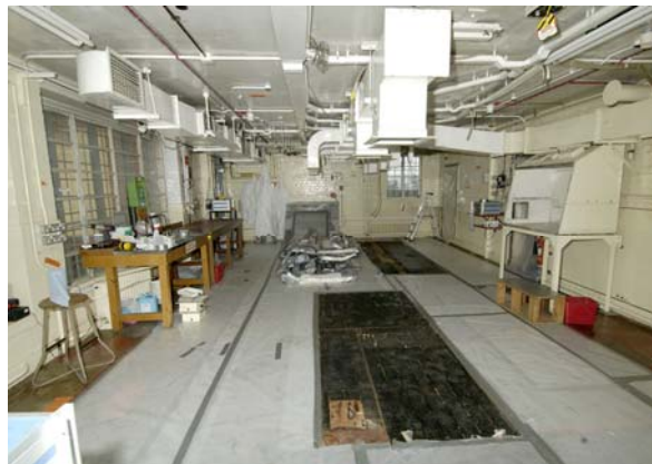
Lab 1 Air-boxes Removed
