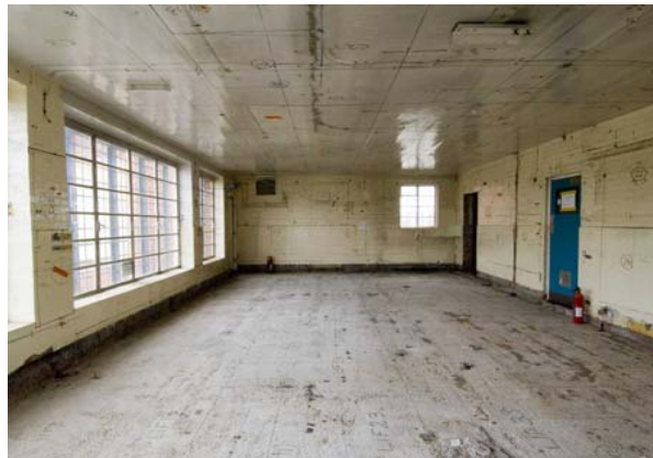
Lab 1 Decommissioning Complete
