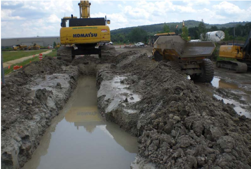
Figure 1. Excavation for the slurry wall.
