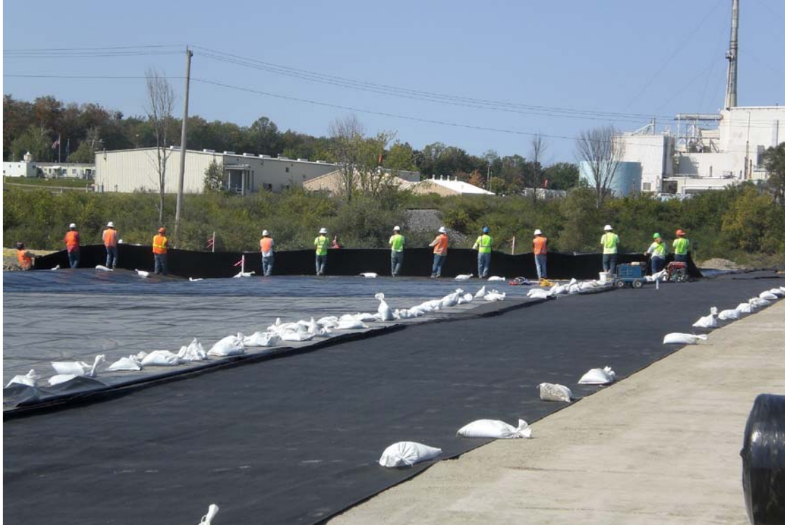
Figure 3. Panel installation in progress.
