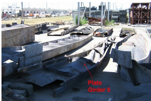
Fig. 4. Girders at the Caltrans storage yard.
