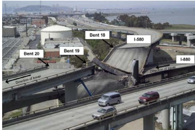
Fig. 2. Postfire aerial view of the collapsed section of I-580 looking west. Picture from Caltrans
