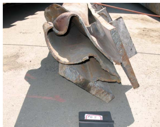
Fig. 5. Photograph of Plate Girder 5 believed to be between Bent 18 and Bent 19.
