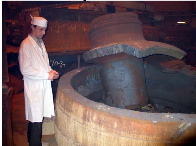
Fig. 4. External view of the HCP tank after partial cutting.
