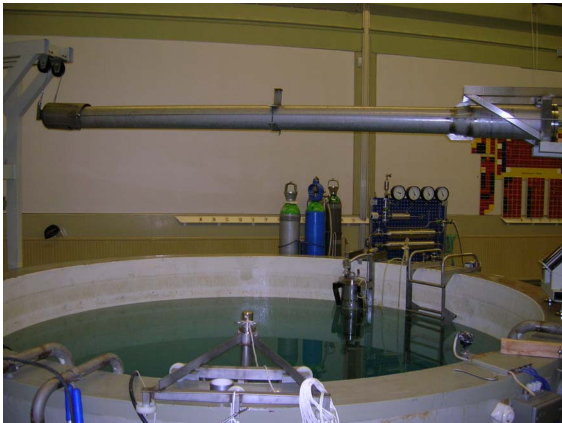
Figure 2 The tilting equipment with the dummy container. The container with corroded fuel is seen at the far side of the pool.
