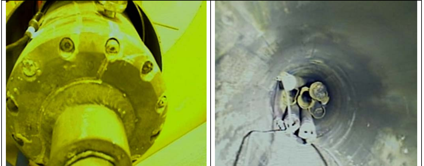
Figure 4: Left: Top of inner canister when the container is removed. Right: Top of the fuel element in the canister when the aluminum top of the 4 corroded rods is removed
