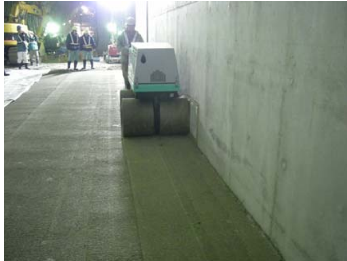
Figure 7. Compaction by small vibrating roller at side areas
