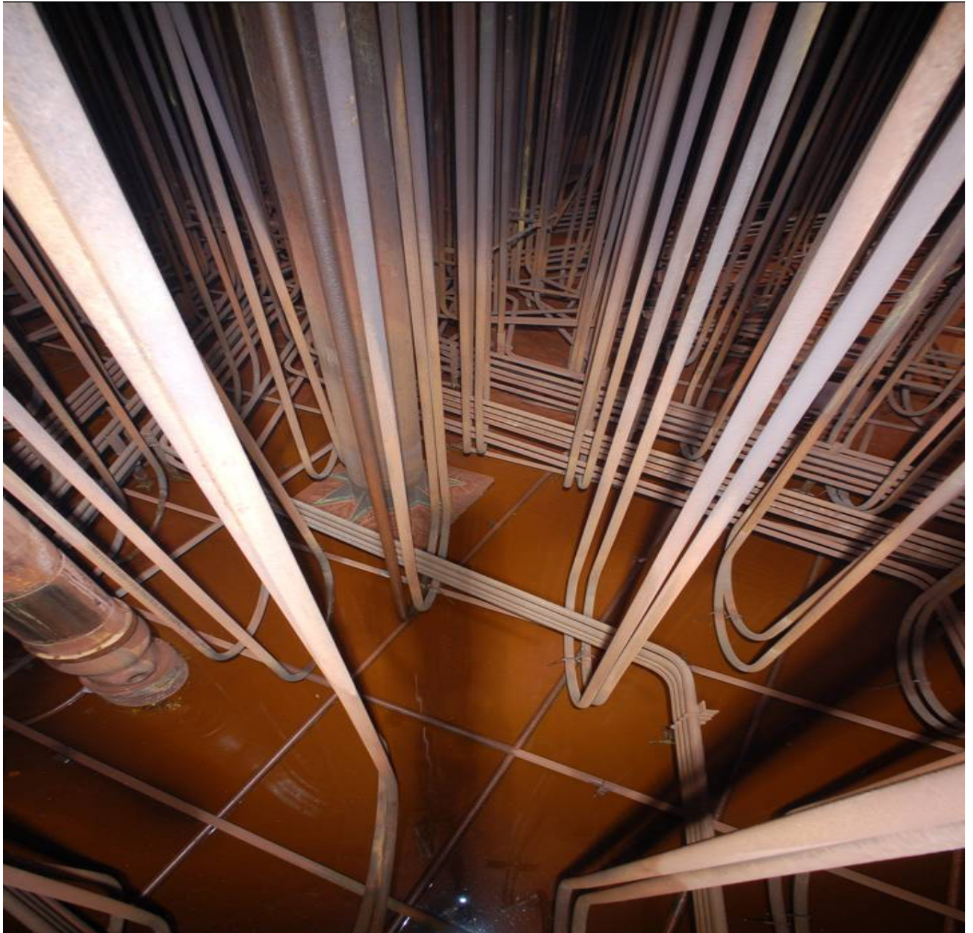
Figure 4. Tank 5 after the second Chemical Cleaning acid strike.
