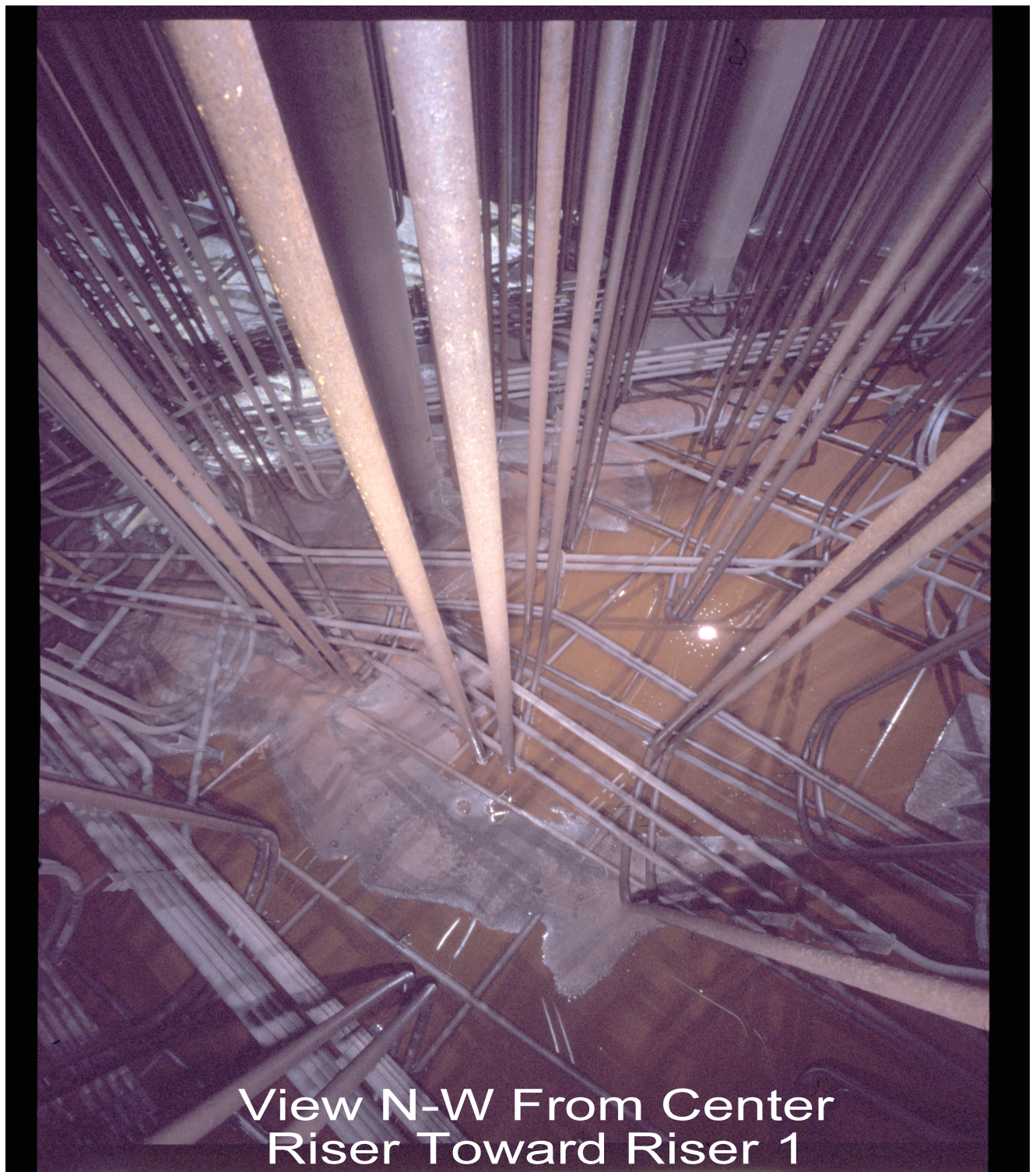
Figure 3. Tank 5 prior to completion of mechanical cleaning.
