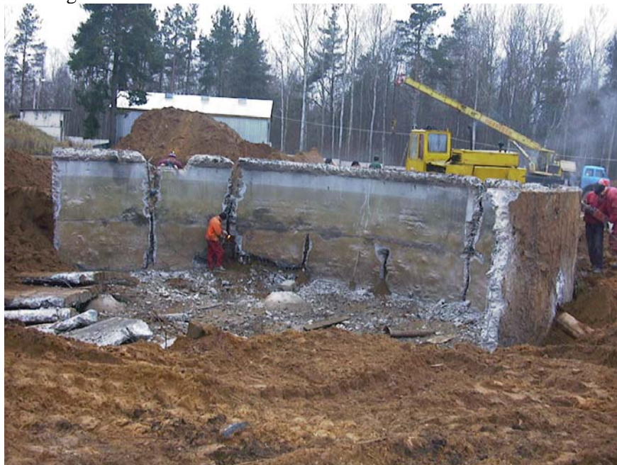
Fig. 4. Dismantling of unused 400 m 3 tank.
