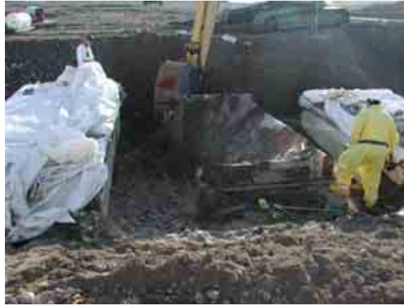
Fig. 3. Typical container condition for early generation retrievably stored wastes
