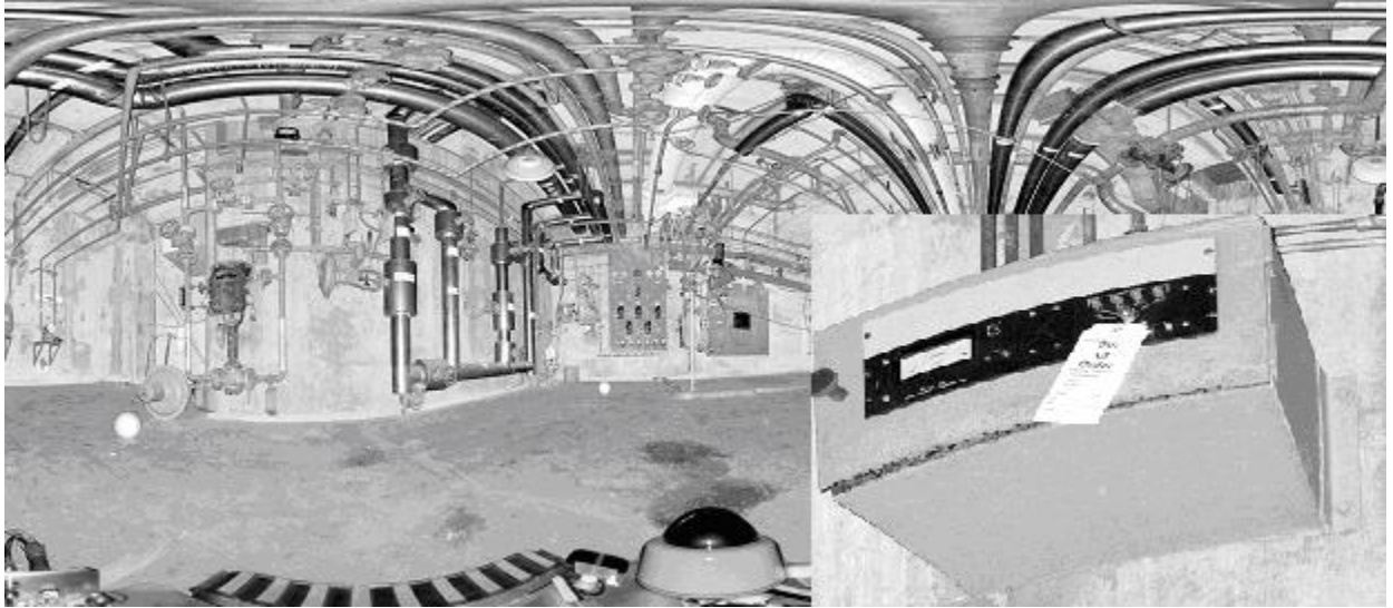
Figure 2. Raw image of a portion of the 105-P Purification Room at SRS. Image has characteristic spherical distortion including the robot on-board camera and robot tracks at the bottom of the image. Insert is a blow-up of one device in the facility.
