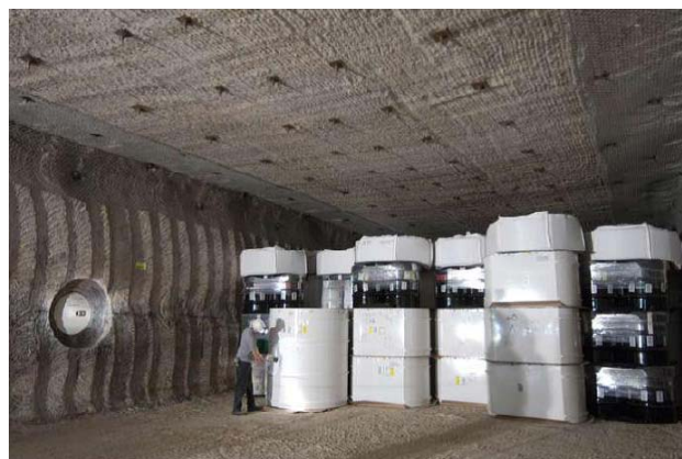
Fig. 3. Over 10,000 nuclear waste drums and standard waste boxes filling 1 of 56 rooms to be filled at WIPP over a 20-year period. Almost 25 rooms have been filled as of June 2008. Note the higher activity remote handled waste plunged into boreholes in the wall to the right and plugged with four feet metal-wrapped cement.
