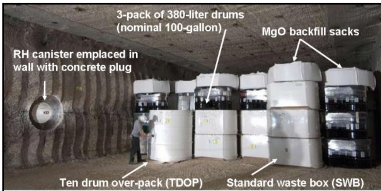
Fig. 1. A previously emplaced RH waste canister has been inserted in the borehole in the wall at left, with a concrete plug in front to shield personnel working in the CH disposal room.
