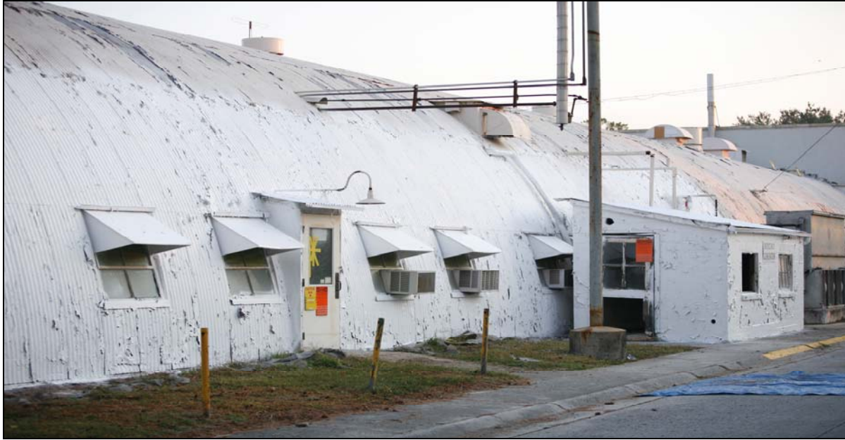
Fig. 3. Building 2000 after PrepLESS PRIMER™ and Your Last Coat™ application
