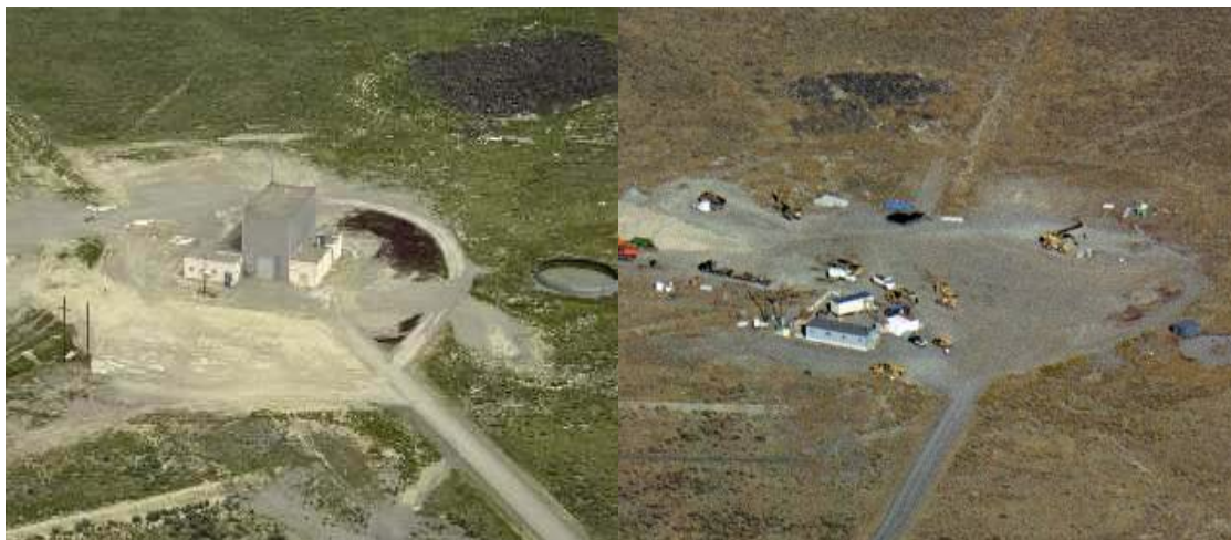
Fig. 3. The Power Burst Facility was demolished 4 years ahead of schedule.
