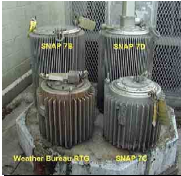
Radioisotope Thermoelectric Generator (RTG) – 700,000 Ci Sr-90
