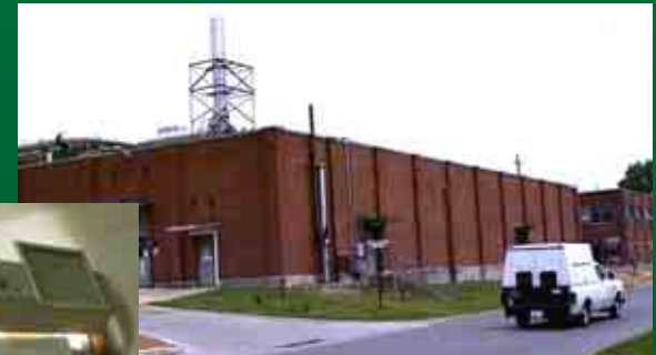
3038 – Radioisotope Laboratory, Alpha Handling Facility
