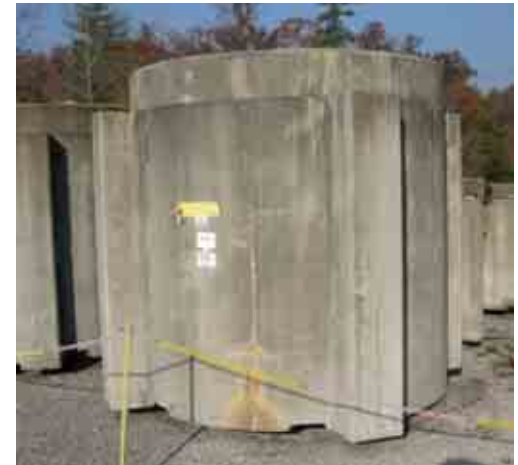
9'x9'x9' concrete vaults used to store legacy RH waste
