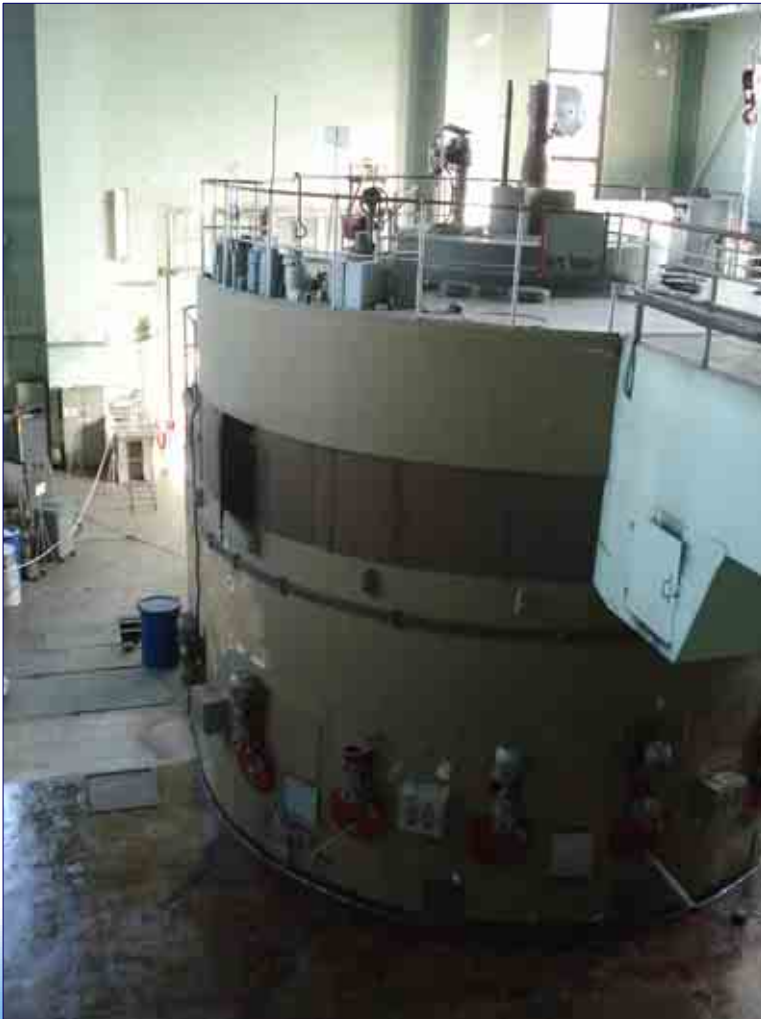
VVR-S Research Reactor, Magurele, Romania
