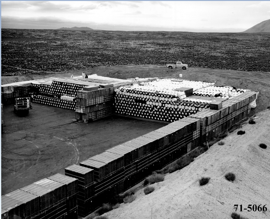
Early placement of transuranic waste storage drums and boxes from Rocky Flats
