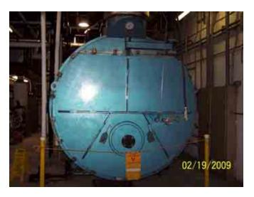
From 40CFR260.10 Definition: Boiler means an enclosed device using controlled flame combustion and having the following characteristics:
