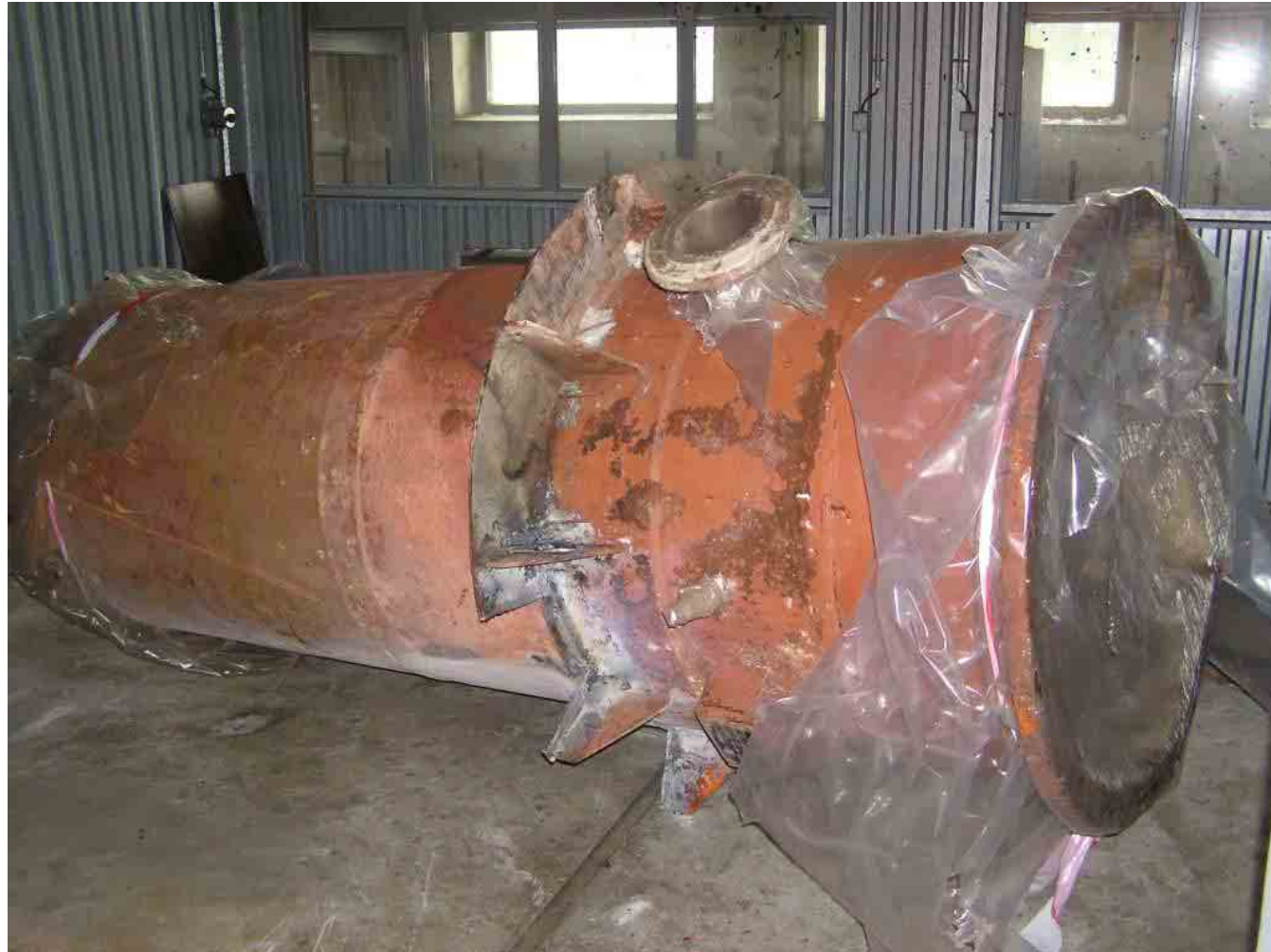
Heater before dismantling
