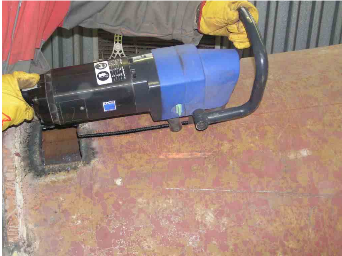
Dismantling with a nibbler
