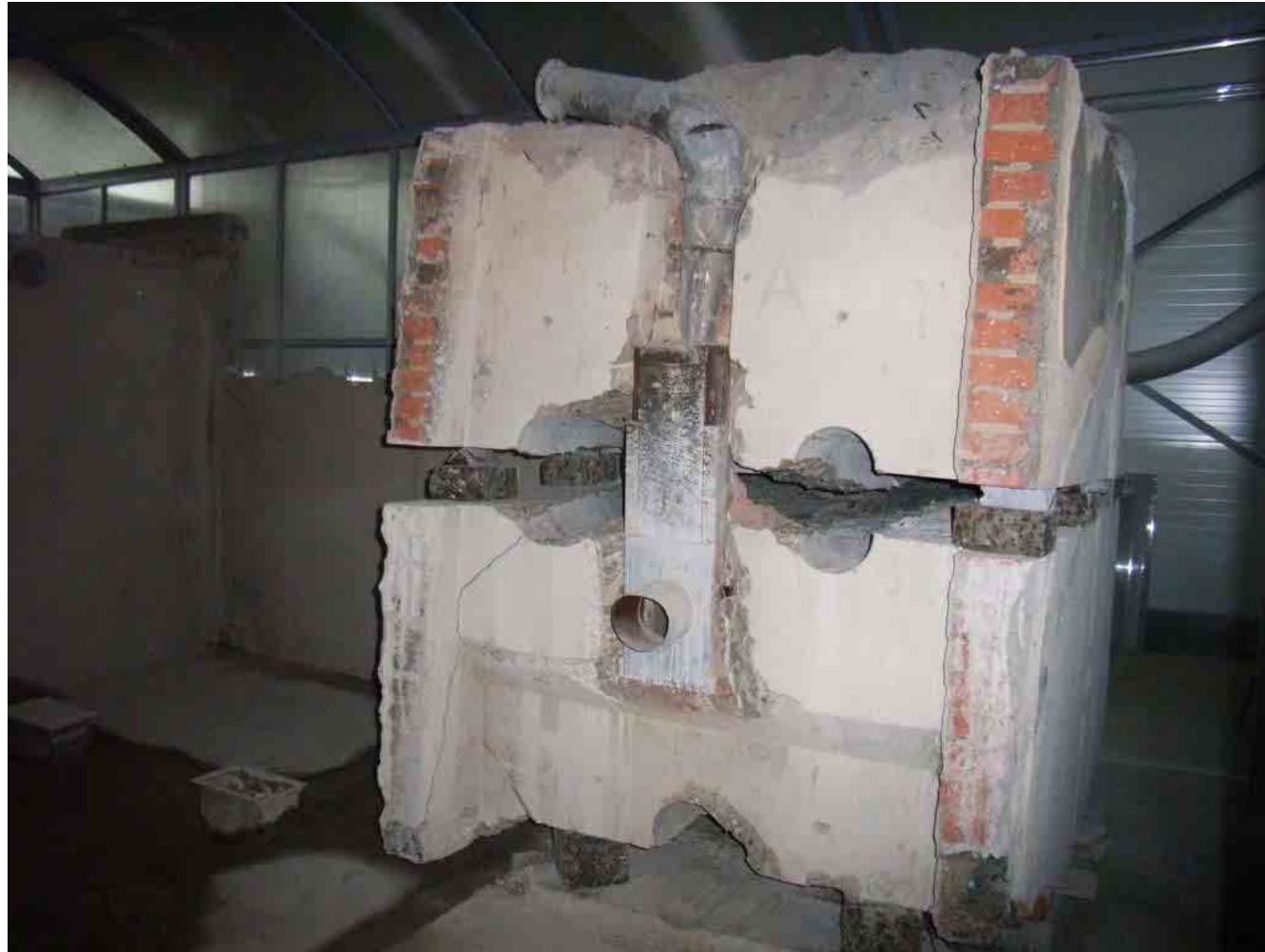
Segmentation of concrete monolith
