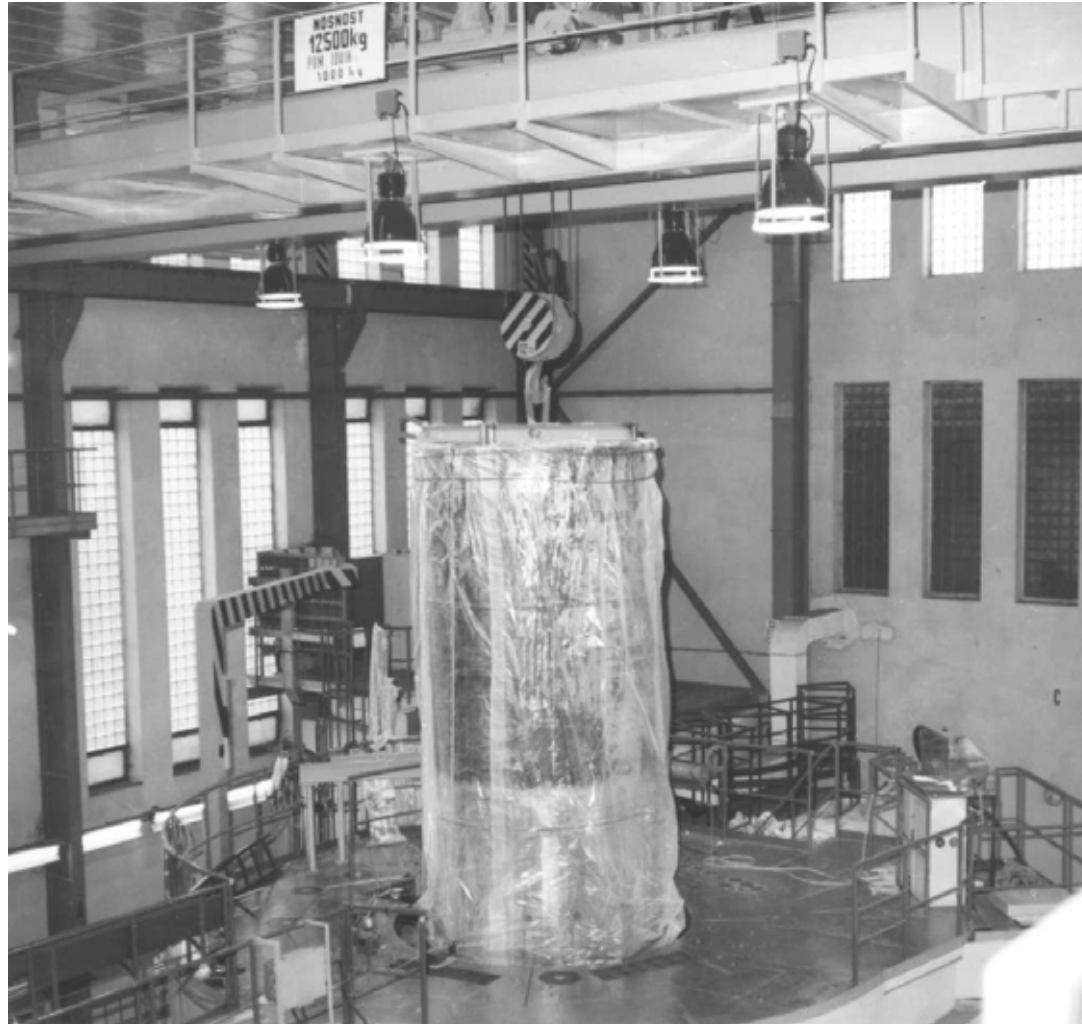
Removing of VVR-S reactor vessel
