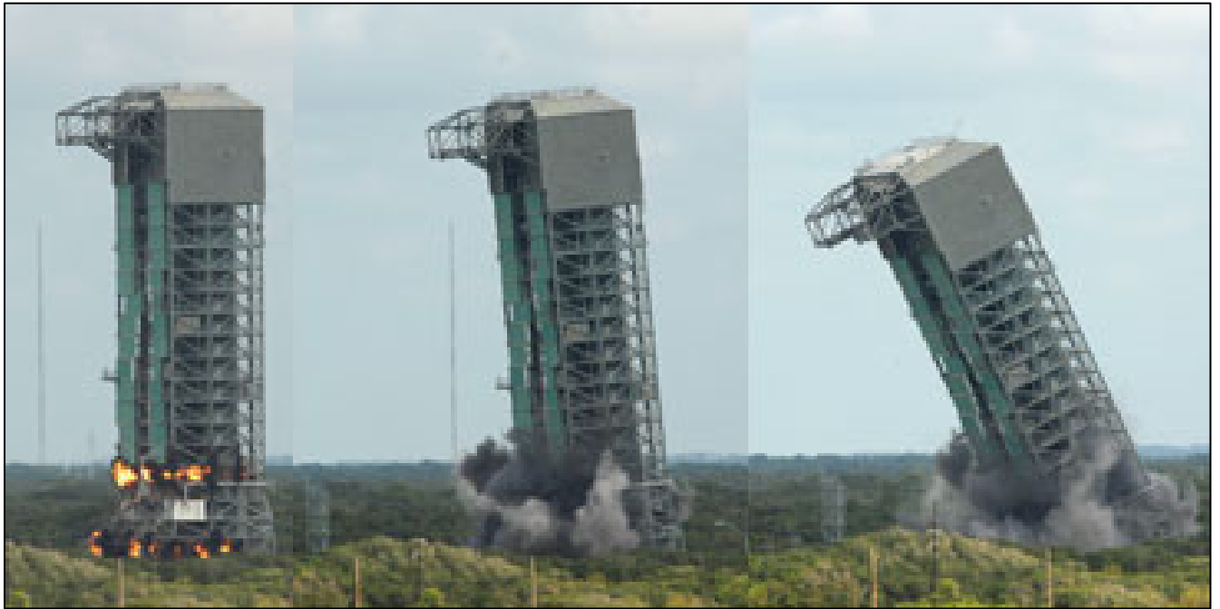
Fig. 3. Atlas 36 MST Sequence of Explosive Demolition.
