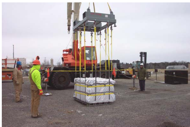
Fig. 6. A loaded bag is lifted by a crane.
