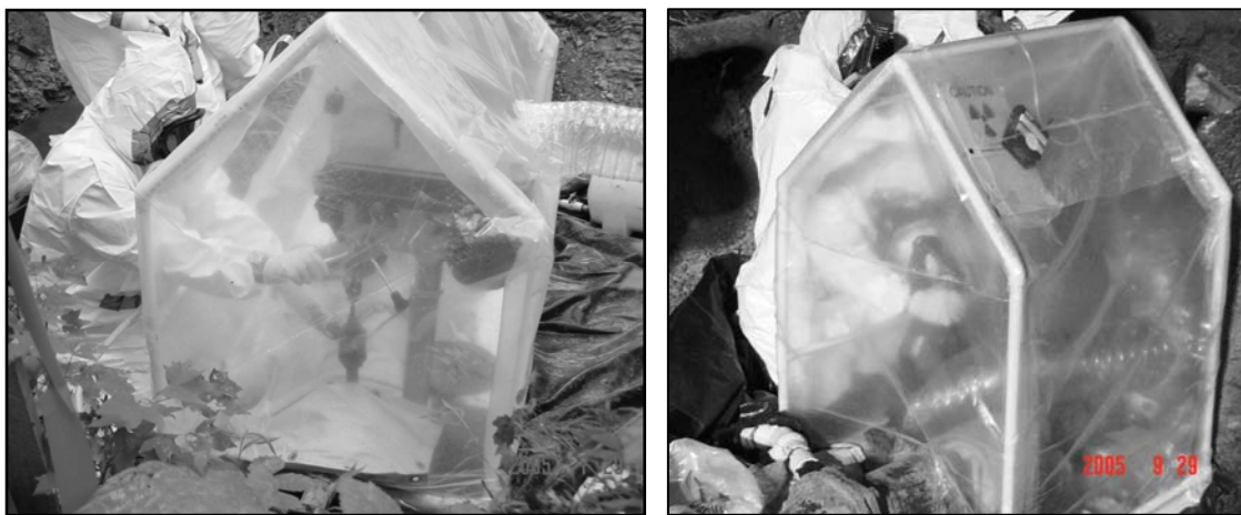
Fig. 4. Tapping LLW Line Using Drill Press ( left ) and Cutting Line With Reciprocating Saw ( right )
