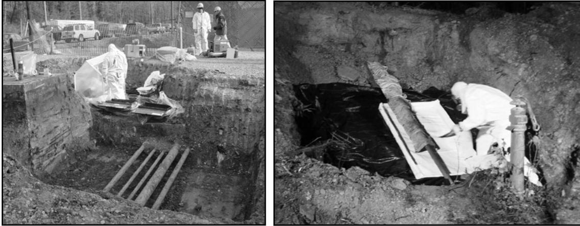
Fig. 2. LLW Pipelines Exposed in Excavations ( left ) and Placing Lead Shielding on Pipeline ( right )
