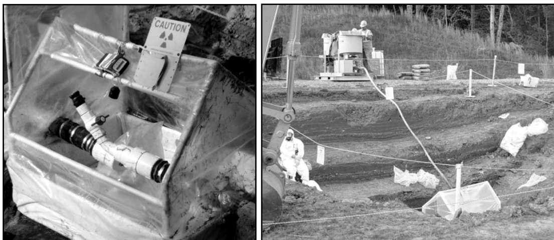
Fig. 3. Grout Fittings ( left ) and Grout Set-Up ( right )
