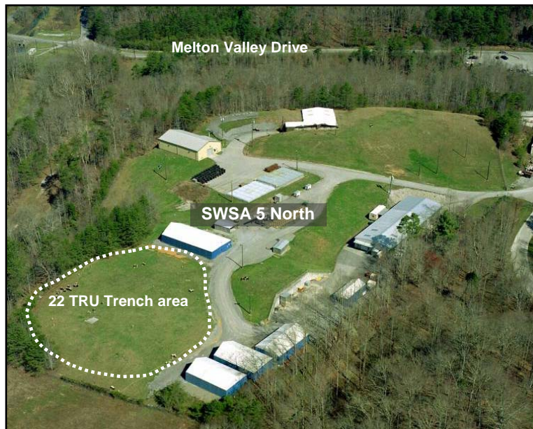
Fig.1 Site Conditions at 22-Trench Area Prior to Retrieval of TRU Waste
