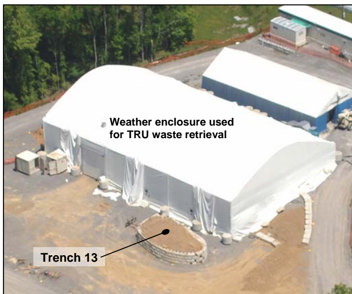
Fig. 4. Photo showing stabilized Trench 13 and the weather enclosure
