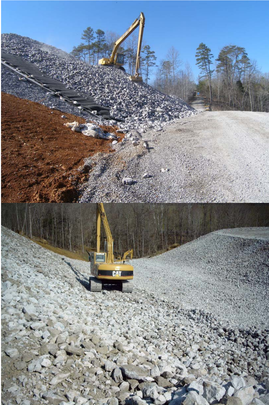
Fig. 4. – Placing of rock buttresses.
