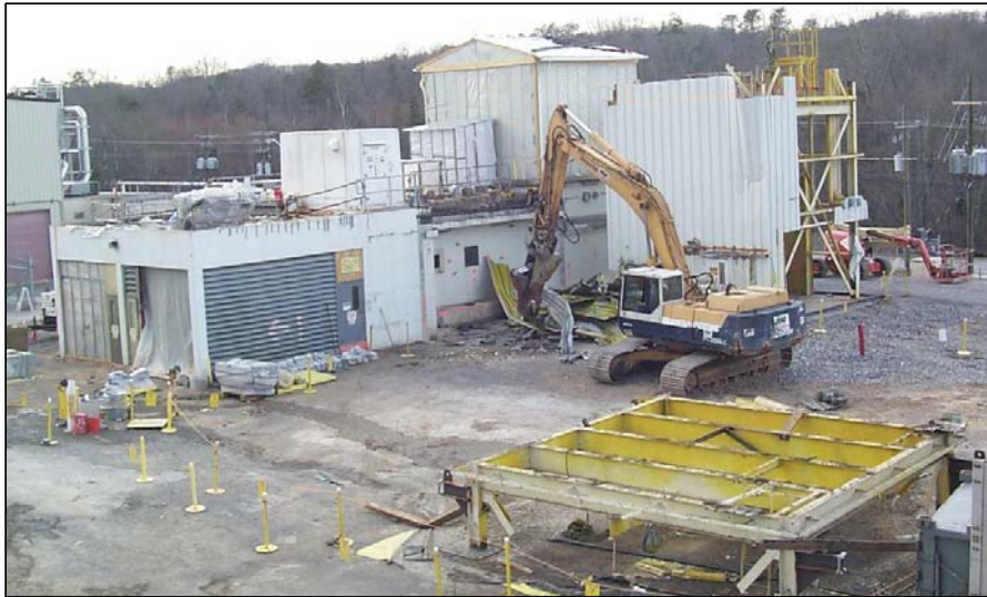
Figure III. Demolition of the Old Hydrofracture Facility.
