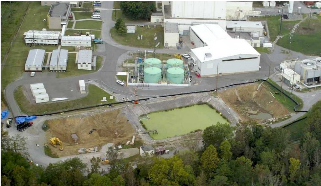
Figure III. Remediation of the HFIR Impoundments.
