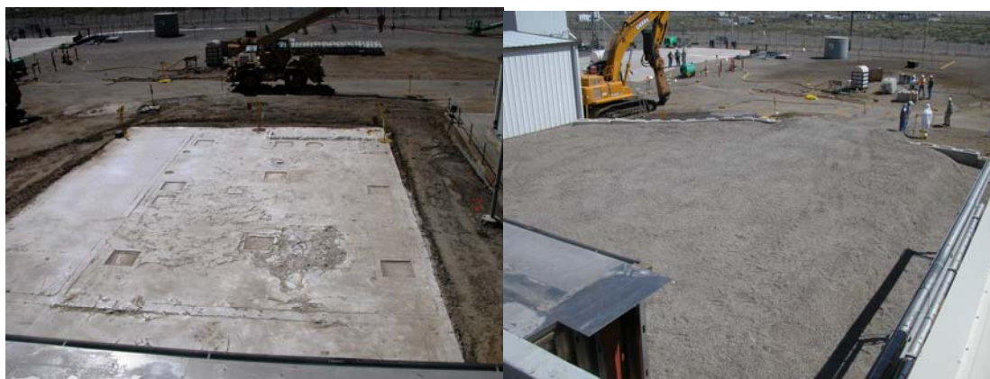
Figure 4. Final Decommissioning End-Point Completion: Clean Slab on Grade
