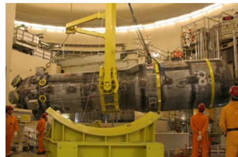
Figure 3 and 4: CLOSING of the openings and dismantling of the Steam Generators
