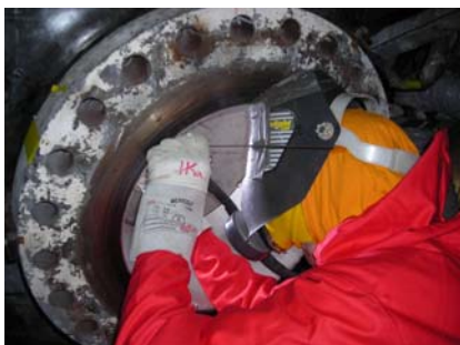
Figure 3 and 4: CLOSING of the openings and dismantling of the Steam Generators
