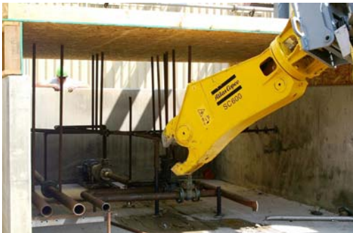
Fig. 3. Pipe shear moving into the vault for cutting piping.
