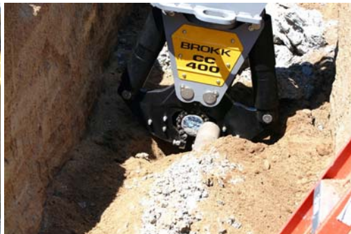
Fig. 4. Pipe joints covered with concrete in the trench mockup.
