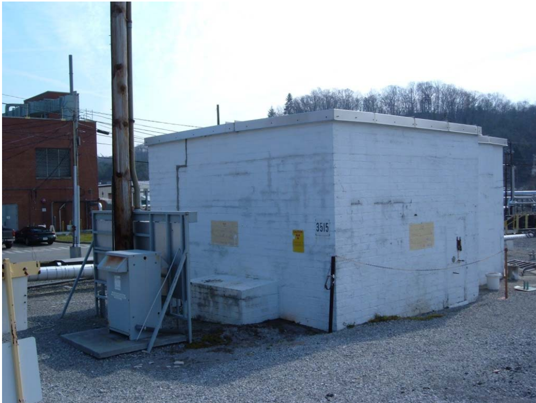
Fig. 1. North and west side of Building 3515.
