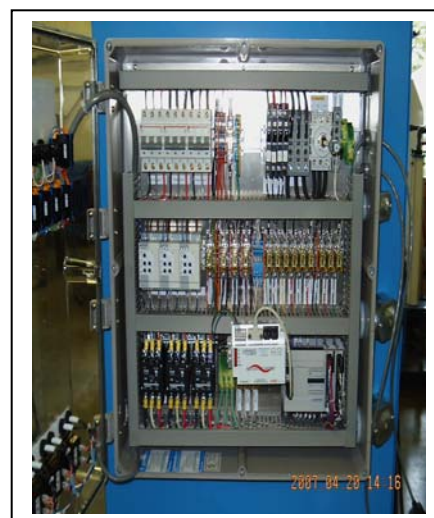
Figure 1. EC Cell Skid (5 gpm each)
