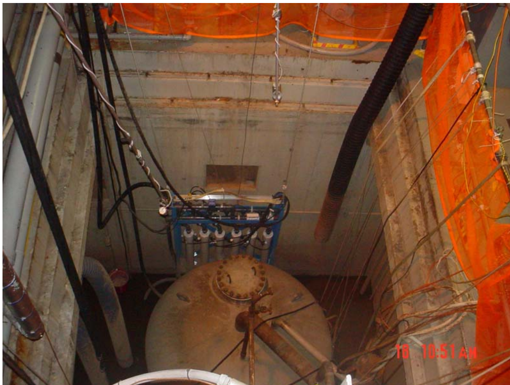
Figure 3. EC Cell Skid lowered into place in demineralizer vault
