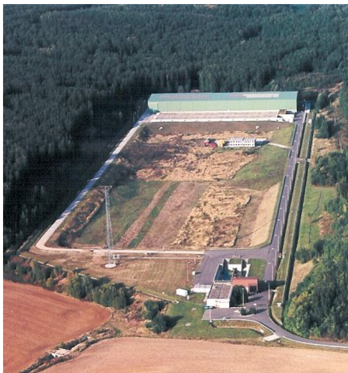
Fig. 1. The National Radioactive waste Repository in Mochovce, Slovak Republic.
