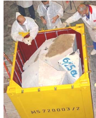
Picture 15: Storing the blocks into Konrad Type-II container
