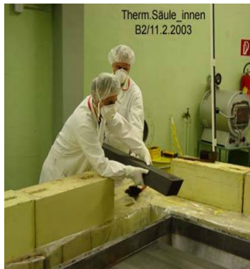
Picture 5: Inner Thermal Column, neutron dose, recovering of the graphite annealing
