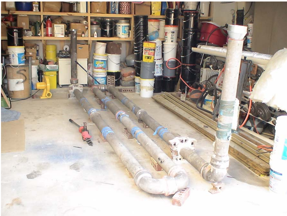
Fig. 2. Pipe test loop after wax treatment and removal of soil
