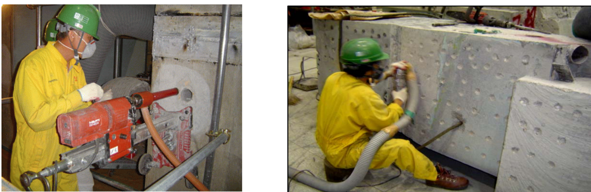
Fig. 7. Sampling from the biological shielding concretes
