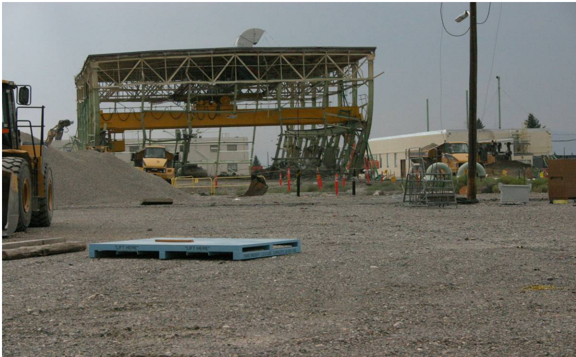
Figure 3. Building TRA-642 pullover
