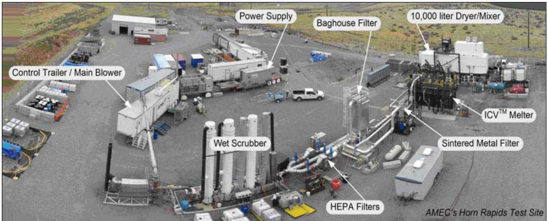
Fig. 3 GeoMelt® full-scale ICV™ equipment.
