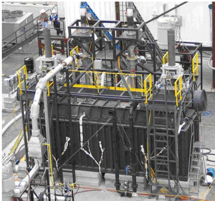
Fig. 3. Full-scale ICV™ test assembly at AMEC's site in Richland, WA.
