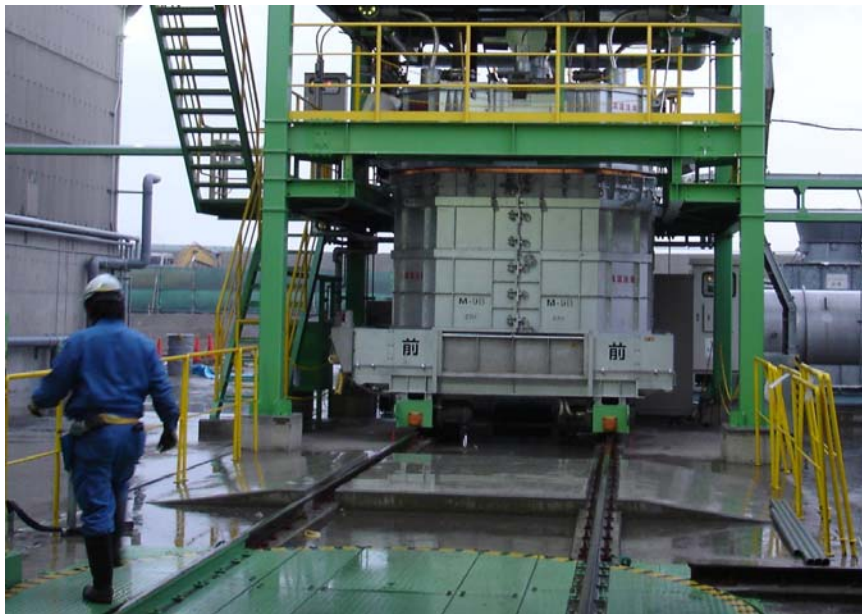
Fig. 3. Rail-mounted melt container during asbestos melt operation.
