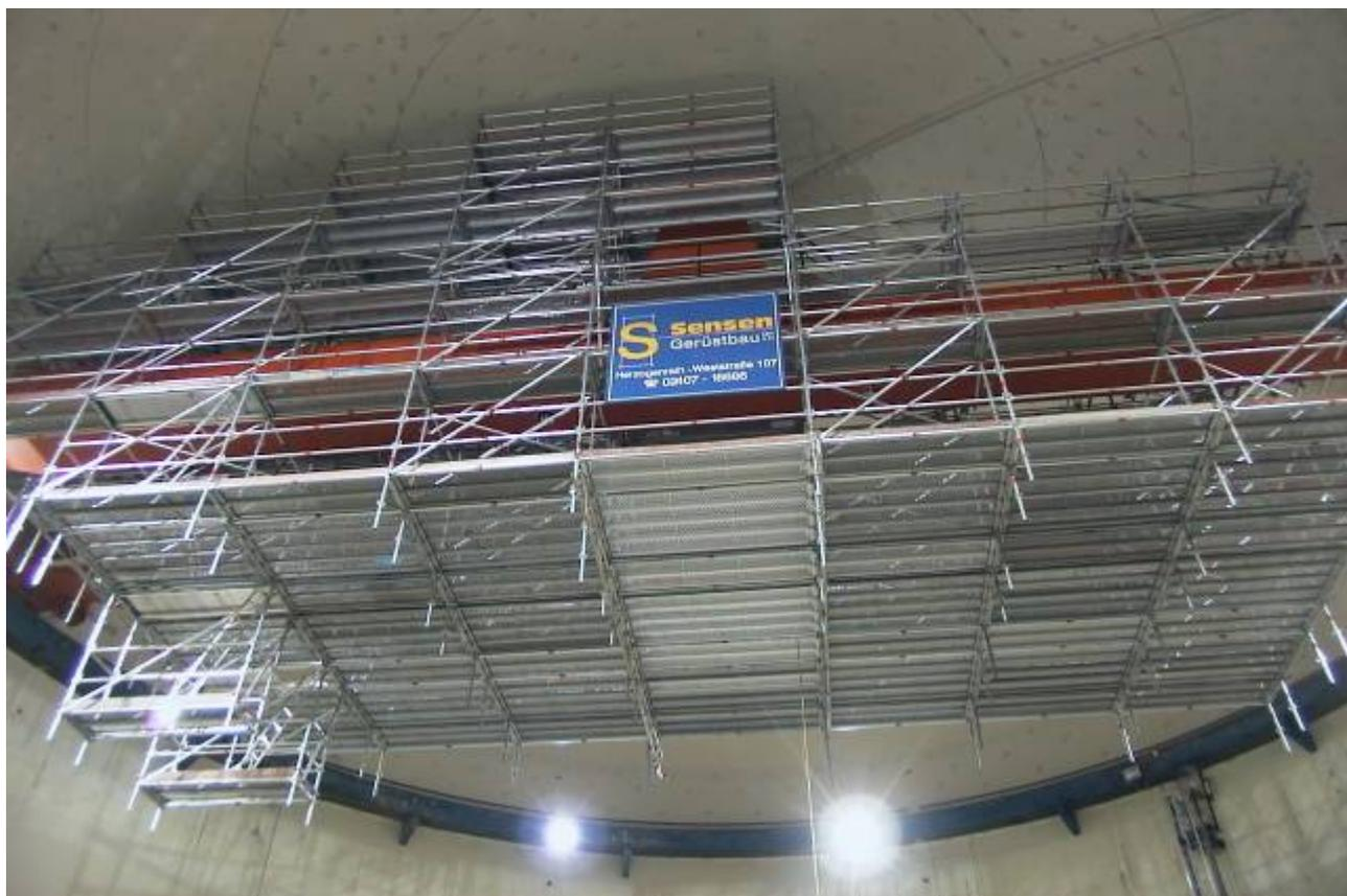
**Fig. 16. Suspended scaffold on 10 Mg hall crane**
