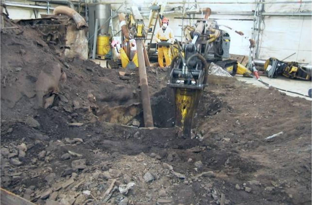
**Fig. 14. Disassembly of the biological shield with disassembly robots and rock chisel**
