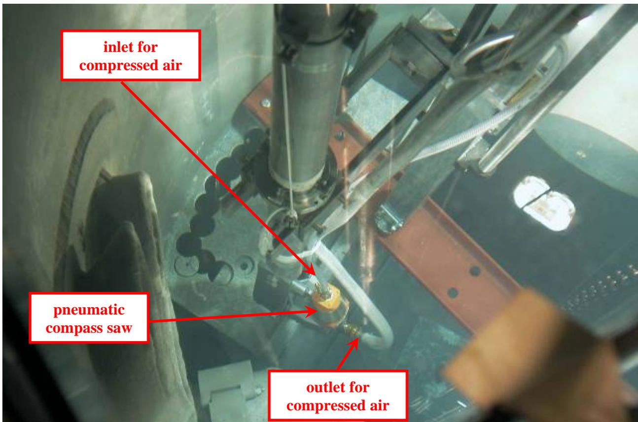
**Fig. 9. Removal of equipment installed in reactor tank – sawing underwater**
