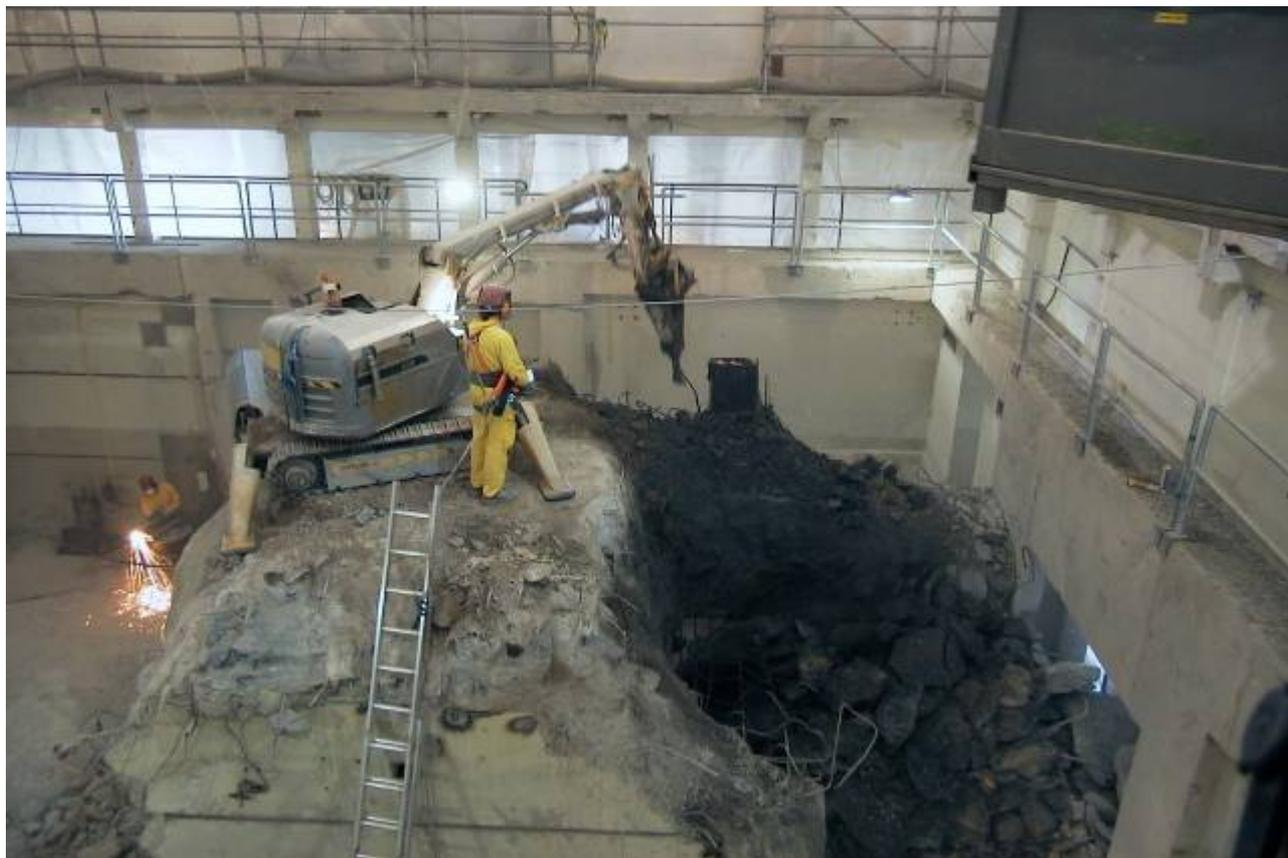
**Fig. 15. Demolition of intermediate ceilings and walls – expanded decontamination**
