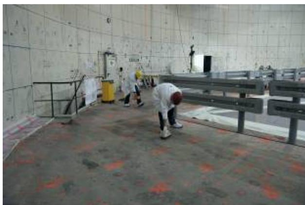
**Fig. 18. Clearance Measurement of floors walls**
