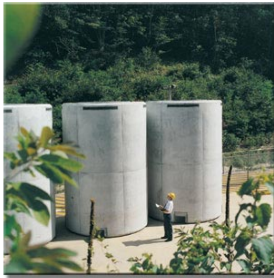
Fig. 4. Concrete casks at Palisades site, U.S.A. ( www.bngfuelsolutions.com )
