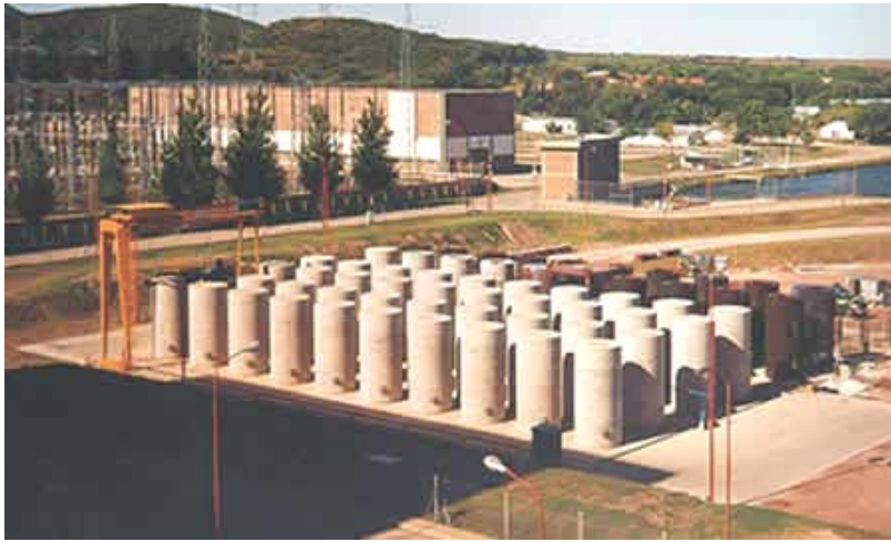
Fig. 2. Argentine storage of SNF placed inside concrete silos (www.invap.net)
