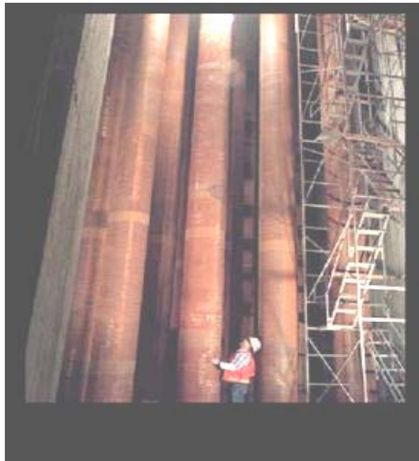
Fig. 1. Metallic pipes view in a vault facility storage type for SNF. (www.qmetrics.com)
